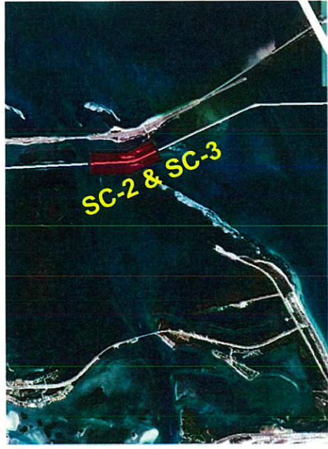
Sunshine Skyway Cuts
